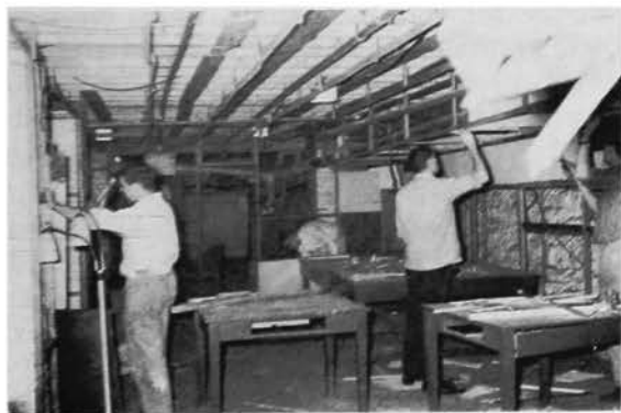
BEFORE: Penn Iotans placing insulation and wall studs to receive the new panels.
