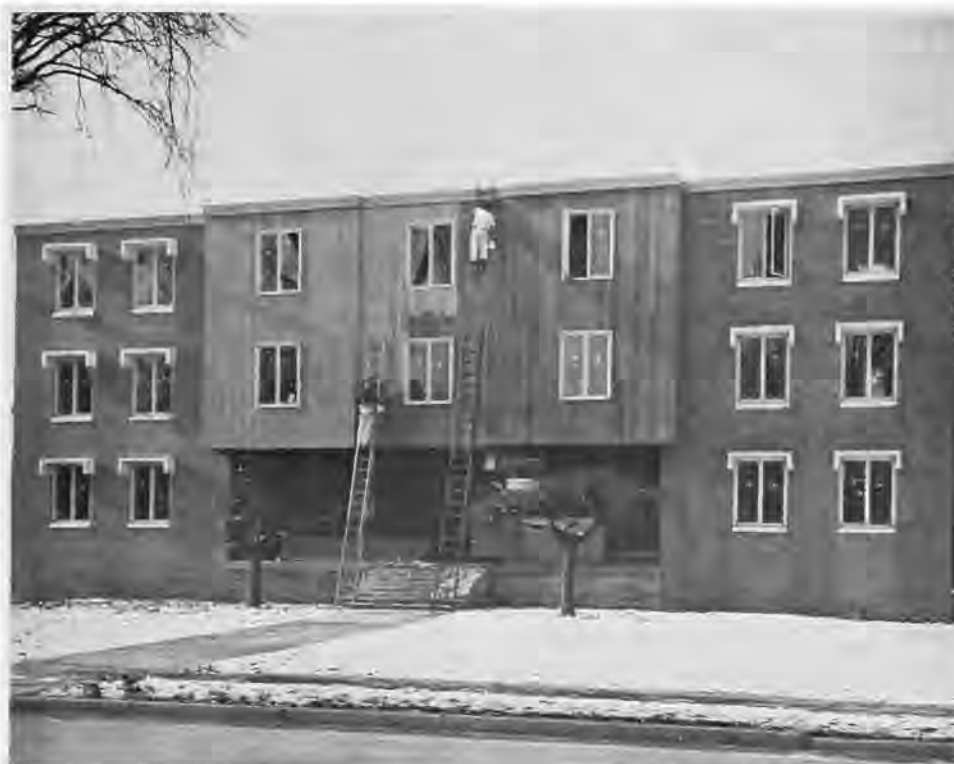
Workmen apply weatherproofing to the redwood front of the rebuilt Phi Psi house at Colgate.
